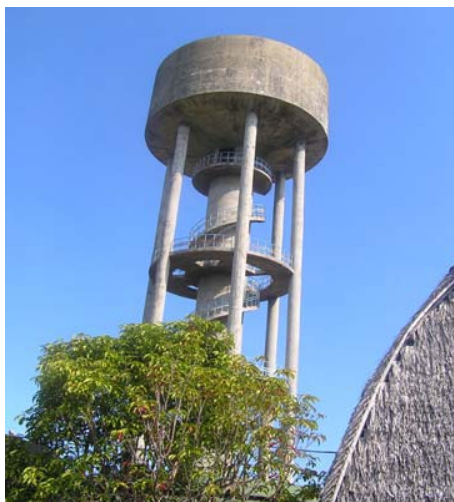
Gambar 3.1a Tower PDAM Jembrana
